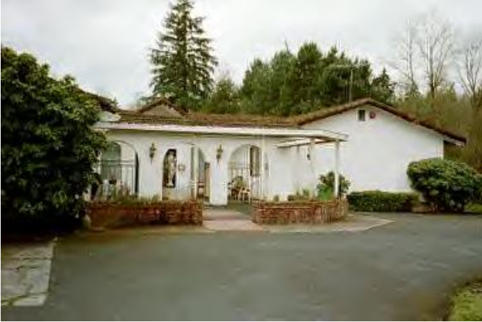
Majdali House in Battle Ground, Washington, USA
